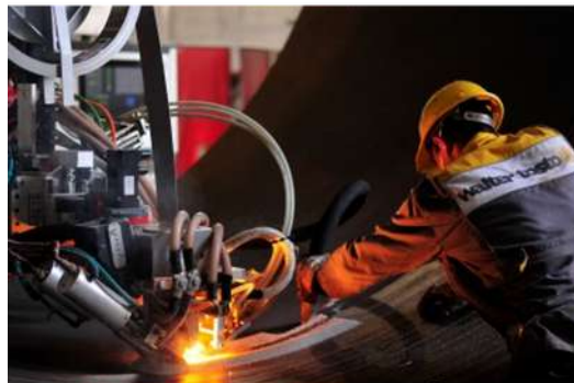
Bottom cladding using robotic GTAW welding
